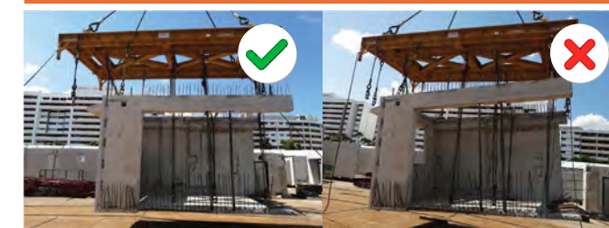
It was a challenge to lift a PPVC module without tilting it
